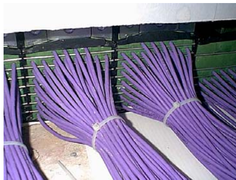
Transit Frame to protect each cable
