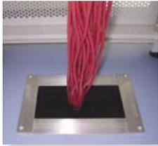
Openings with a large number of cables can be effectively sealed using KoldLoK or CoolControl.
